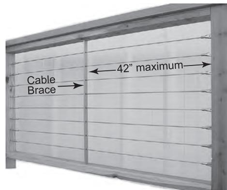
As indicated above, this support can be provided with intermediate posts or a lighter material acting as a cable brace. As with an intermediate post, a cable brace also runs between the top rail and the lower mounting surface, but its purpose is only to support the cable. It is not intended to be an element providing structural support to the railing.
